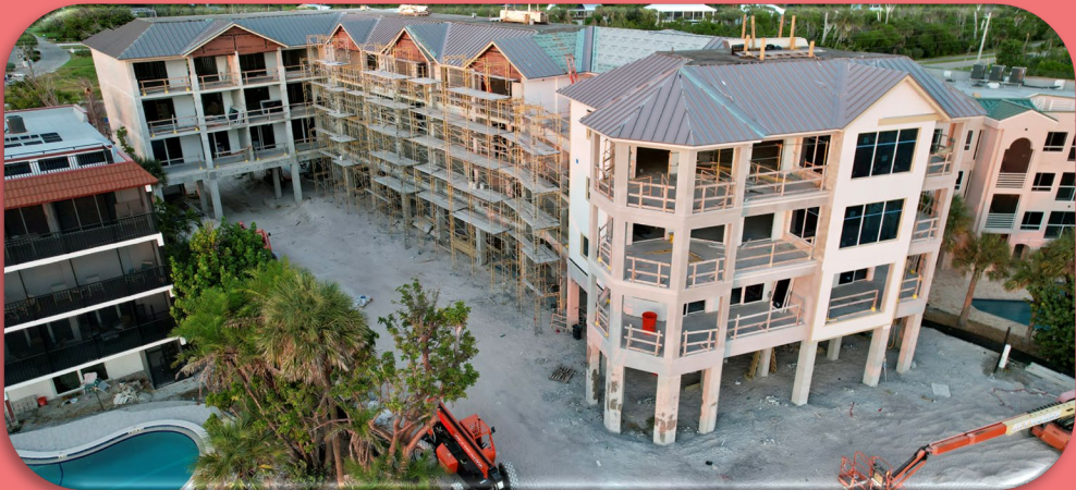
Beachview Villas Construction as of Oct. 24, 2025
